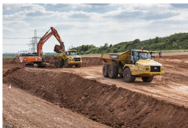
Example of cutting works
