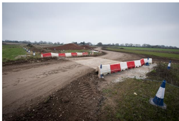
Example of a new haul road in Swinfen
