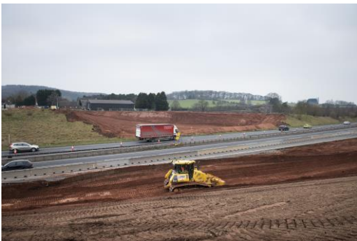
Preparatory works showing where we will build the A5 bridge to enable the railway to pass under the A5
