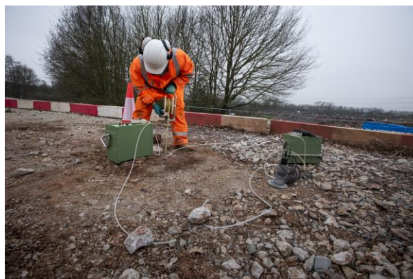
Example of ground investigation works
