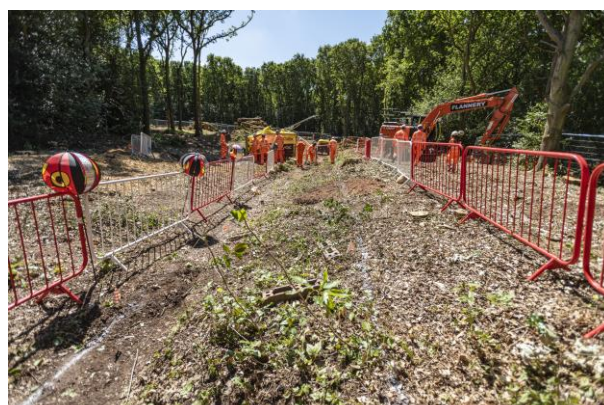
Our team carrying out groundworks
